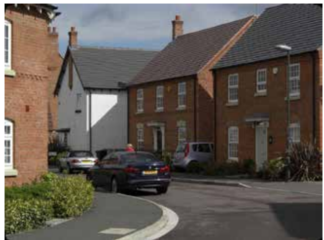
The kerb on this street helps accentuate different functions of the street.
