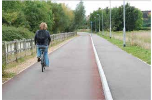
Off-highway cycle track and footpath separated by level and contrasting material with good quality surface and lighting
