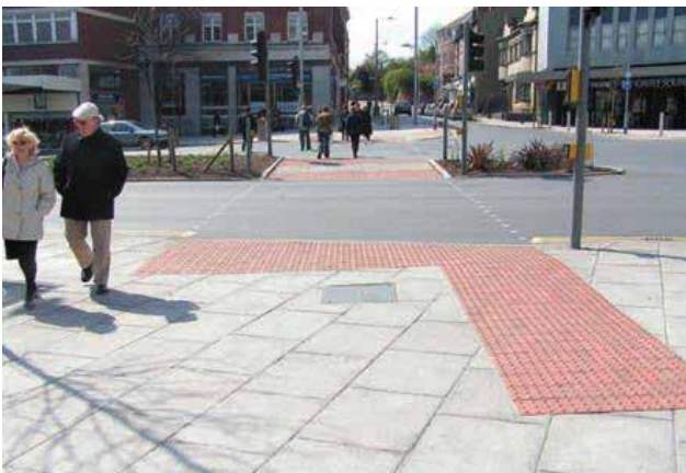
Directly-aligned two-stage pedestrian crossing at Maid Marian Way, Nottingham
