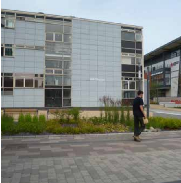
Figure 66 Linked rain gardens on Mill Lane
