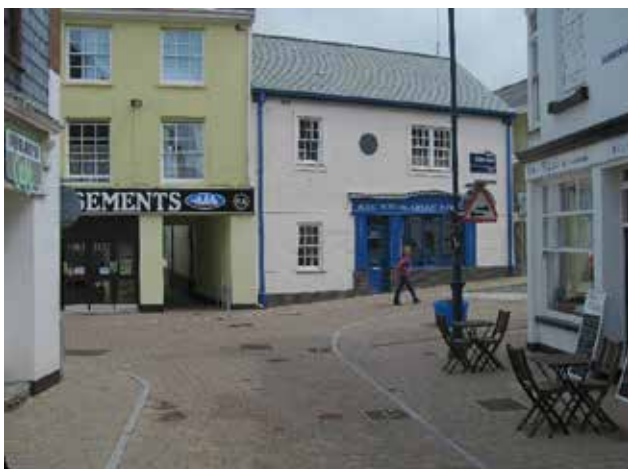
Informal junction in low-traffic retail area
