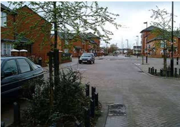
Figure 121 Home Zone in Castle Vale, Birmingham
