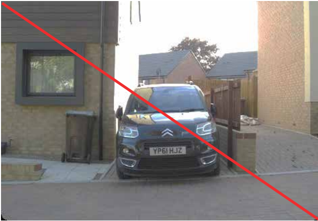
This off-street parking space is ineffective as the car doors cannot be opened.
