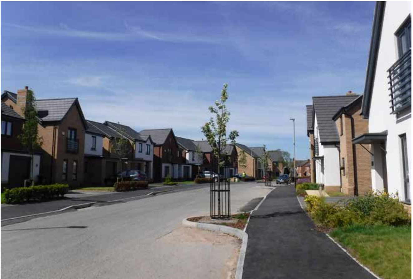
Figure 124 Trees planted in the highway at Ashton Green, Leicester, help to reduce vehicle speeds
