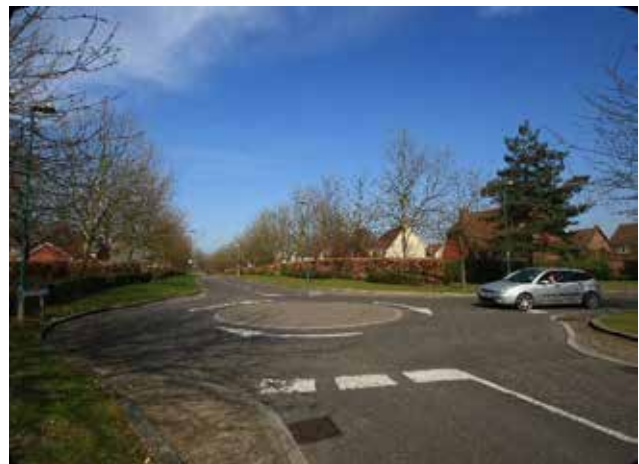
Standard mini-roundabout with overrun areas.
