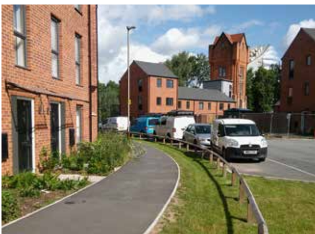
Figure 109 Swale adjacent to the footway at Sock Island, Leicester
