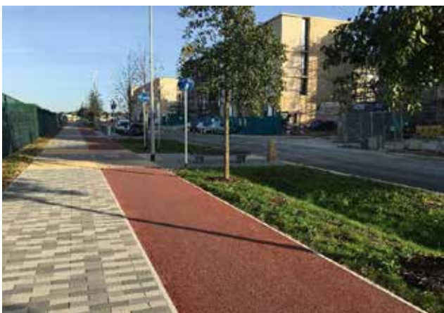
Figure 113 Off-carriageway one-way cycle track through new development, Cambridge
