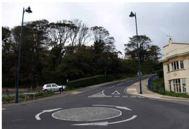
Standard mini-roundabout with textured surfacing
