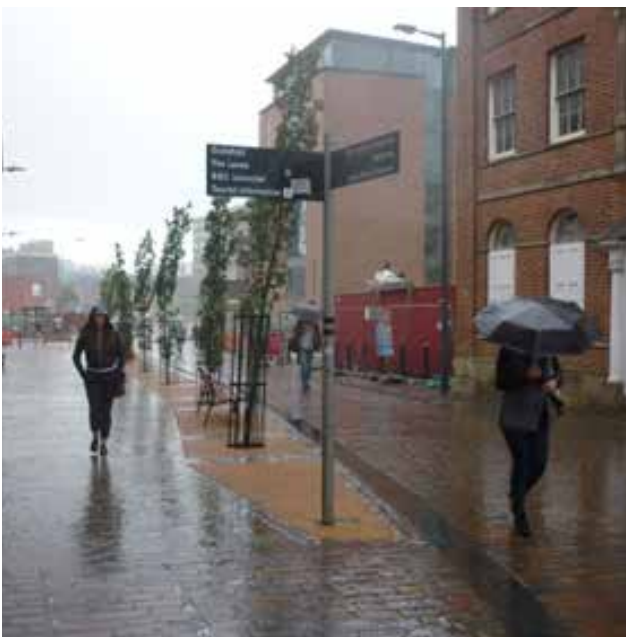
Figure 67 Permeable resin bound-surfaced tree pits on Applegate
