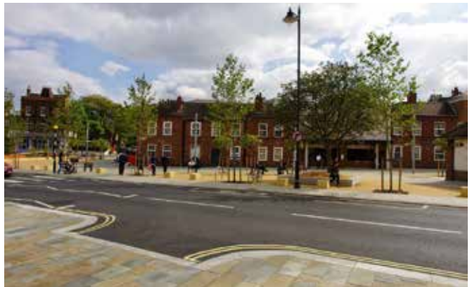
Figure 127 Continuous footways in Clapham Old Town, London
