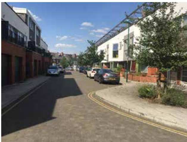
Conventional Street with build out, defined car parking bay and street trees.
