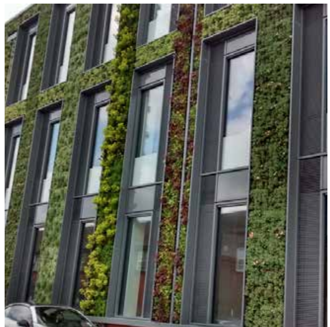
Figure 69 Living wall at University medical sciences building
