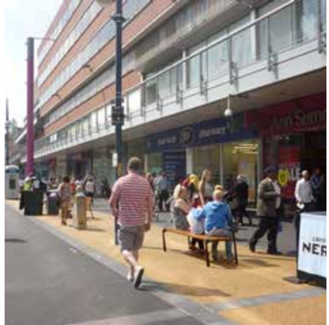
Figure 68 Permeable paving on Humberstone Gate
