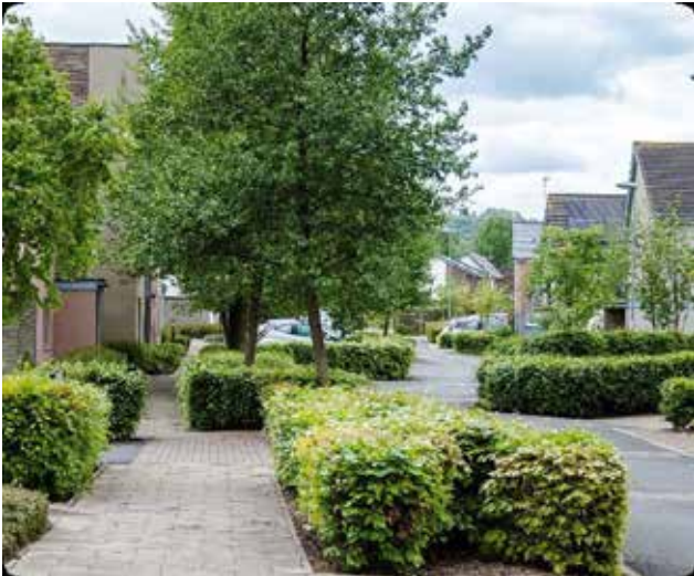
Speeds in this development are limited through design and layout. Alignment, width and landscaped verges are key components.
