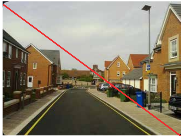
Wheelie bins limit the use of footways, especially by people with disabilities and people with pushchairs. These problems should be eliminated through the design.
