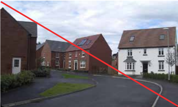
A bend where the generosity of the forward visibility will tend to encourage excessive speed
