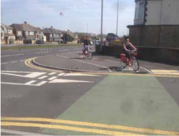
Bent-out crossing, Leeds (Image used under Creative Commons licence CC- BY-SA 3.0, from Cycle Streets photo map: www.cyclestreets.net/location/89767 )
