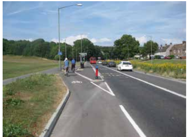
Bus Stop Bypass, Brighton
