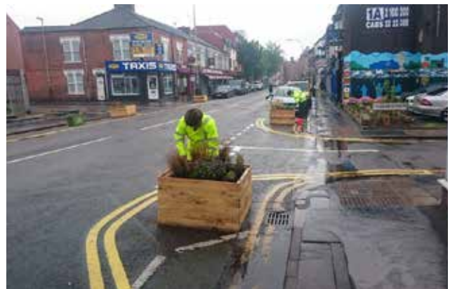
Figure 72 Planters as interim buildouts on Braunstone Gate, Leicester
