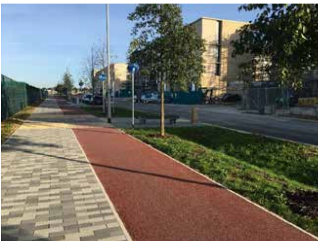
Principal street through new development, Cambridge - off-carriageway one-way cycle track separated from the carriageway by a swale
