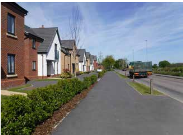
Figure 107 Well defined street at Wheatsheaf works, Leicester
