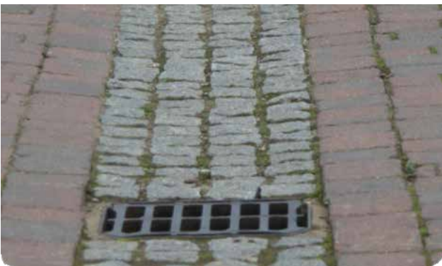
Drainage channel and gully in the centre of a carriageway
