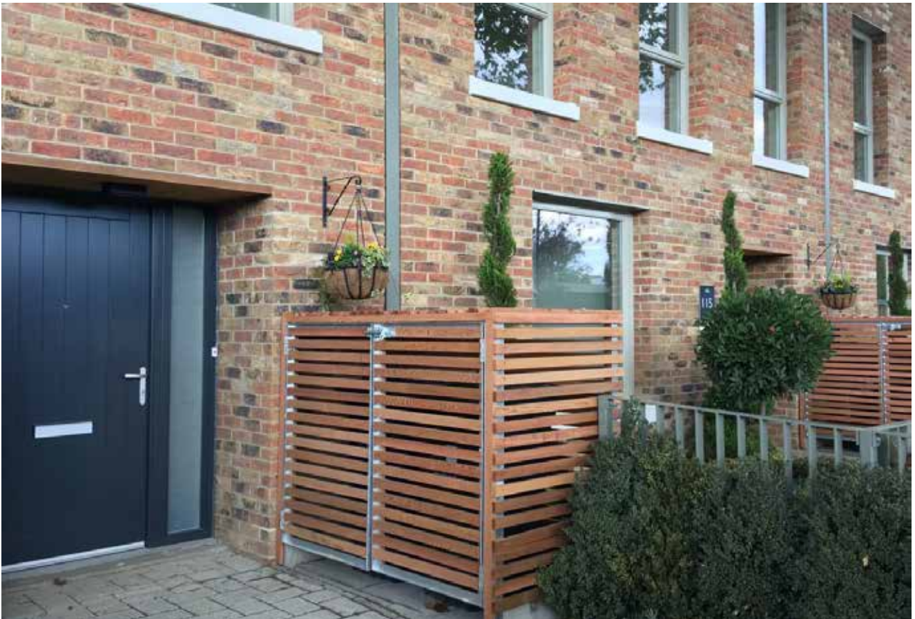
Figure 116 Well designed integrated bin storage
